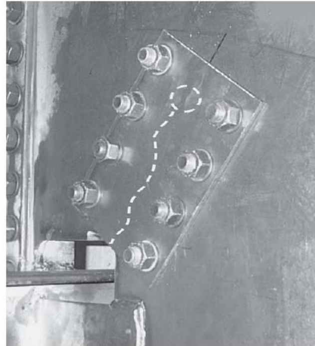
FIGURE A10 Bolted doubler plate repair. Dotted line represents crack line beneath doubler plate and circle is the hole drilled at crack tip to intercept further growth.
