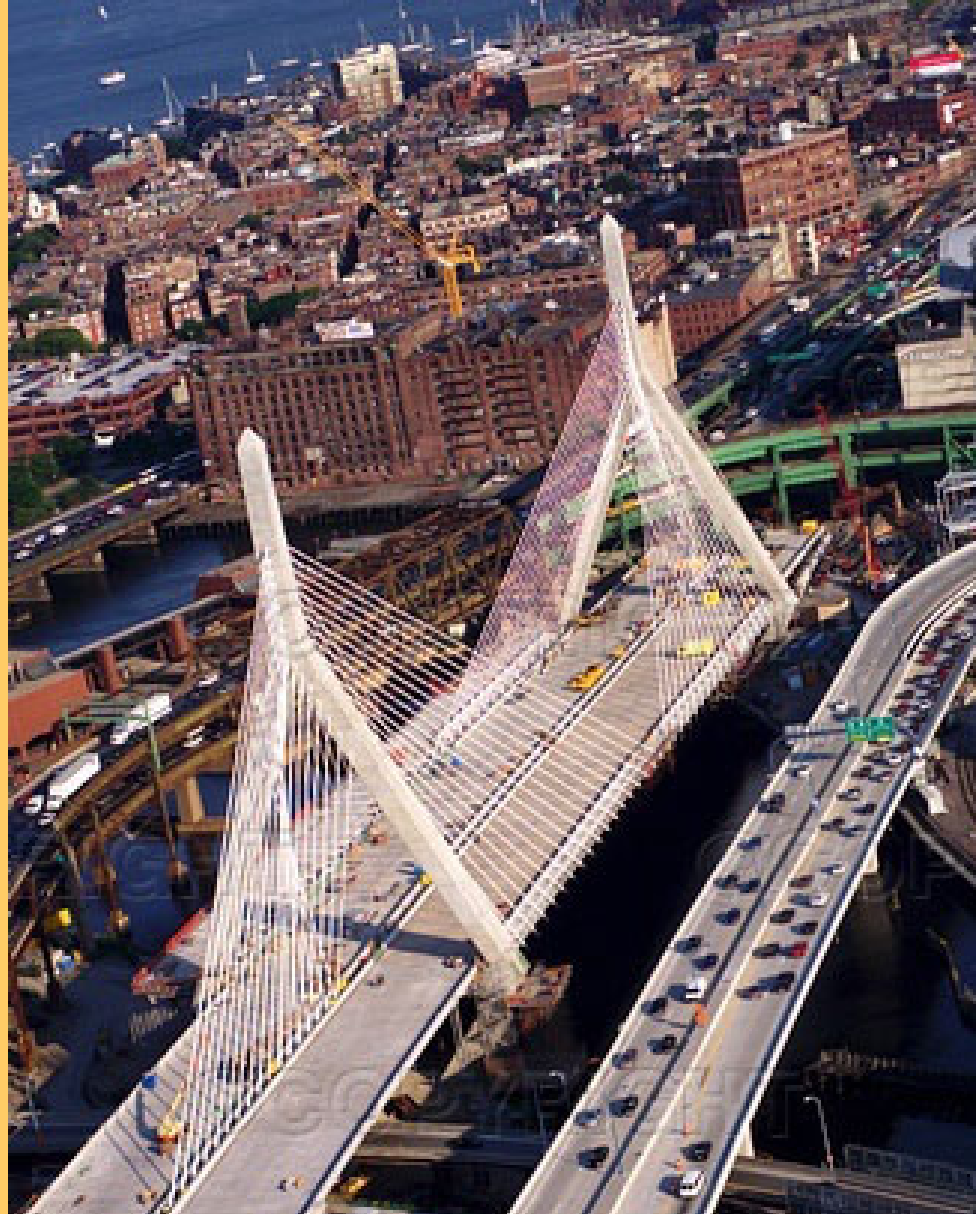
Replacement: Leonard Zakim Bridge, Boston $115M
