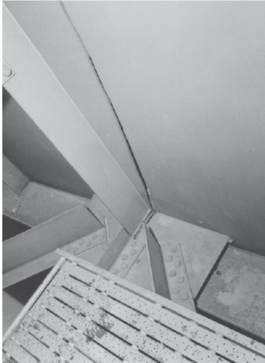
FIGURE 16 View of cracked girder in two-girder span of Lafayette Street Bridge in St. Paul, Minnesota, as an example of a bridge that is sufficiently redundant to avoid collapse despite a fracture of the tension flange and the web of one girder.
